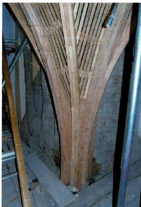
New timberwork for plaster vault
