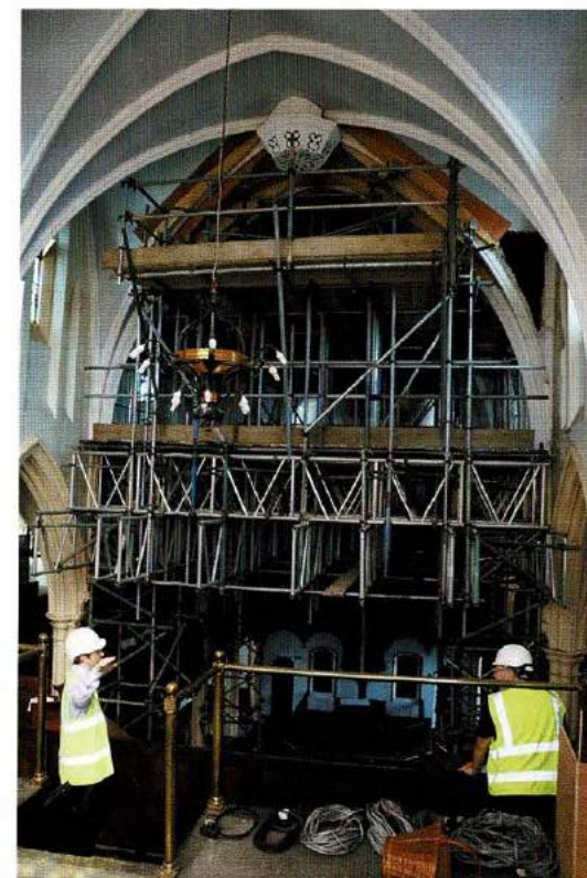
Supporting scaffold to plaster ceiling
