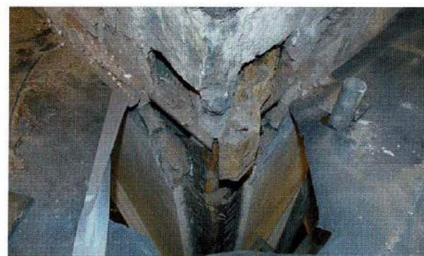
Original timber support to plaster vault springing point
