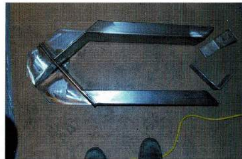
New stainless steel support to plaster vault springing point
