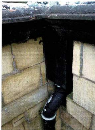
Original gutter let into masonry
