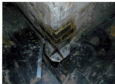
Vault support installed
