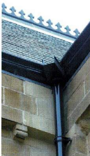
New gutter and chute installed
