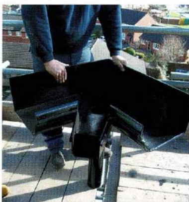
New cast iron gutter corner with chute
