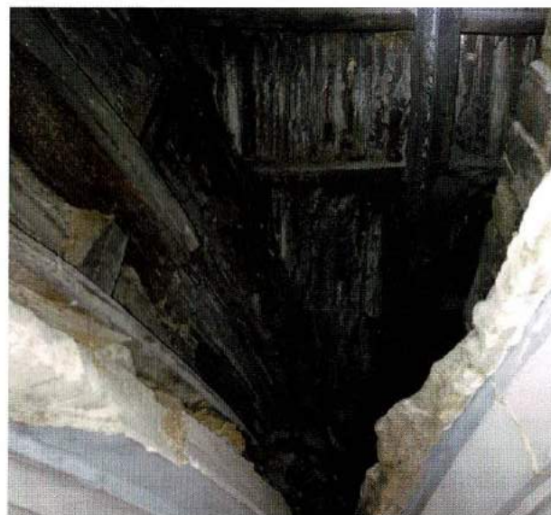
Interior of vault; complete loss of timber rib and laths
