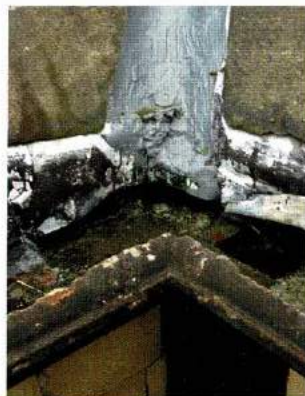
Original gutter intersection and outlet
